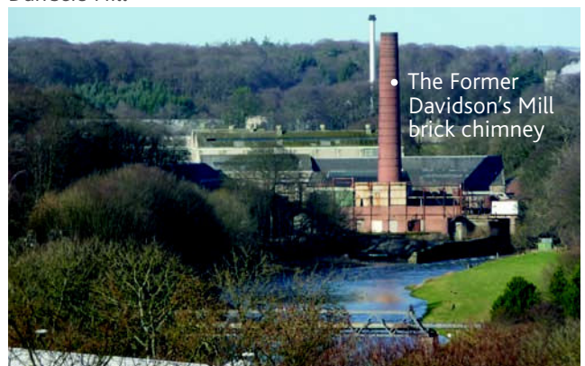
Looking north west towards the site from Auchmill Road
