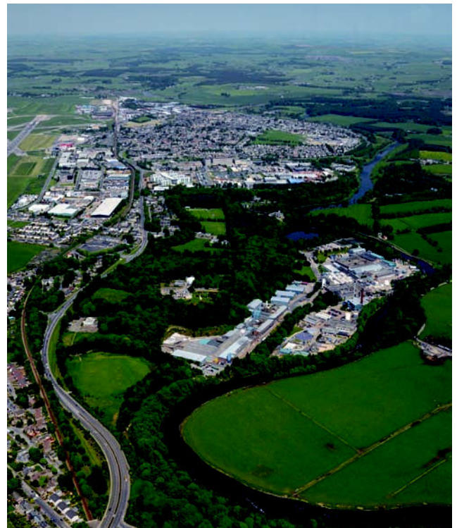
Site aerial photo
